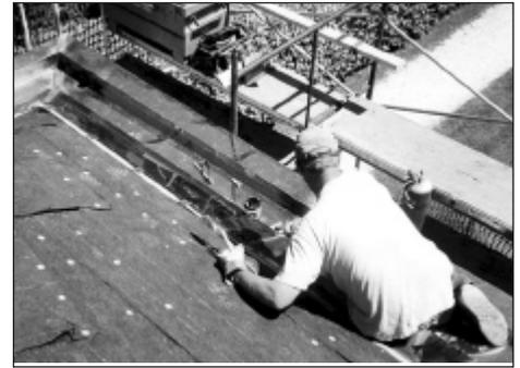
Workers replaced the slate roof and copper gutter and flashing components as part of their duties at the Arlington House Museum
