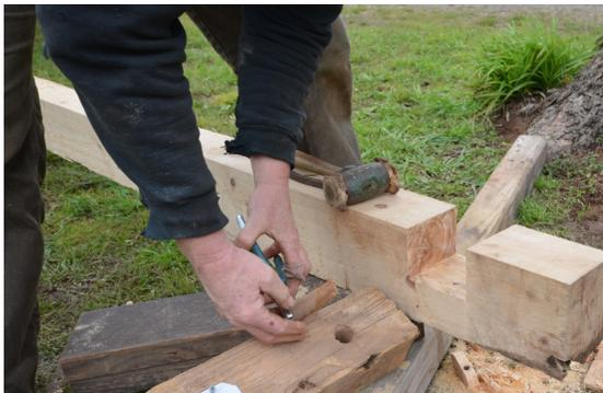
*Example of timber framing joint.*
